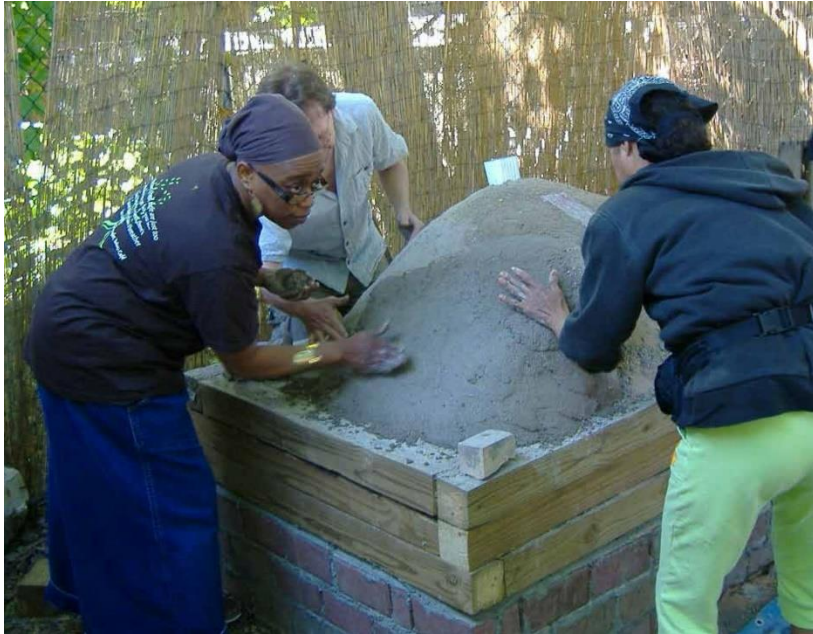
CONSTRUCTION OF CLAY OVEN
